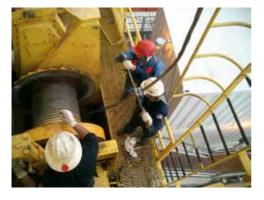
Fixing the rope at the anchorpoint of the drum:
