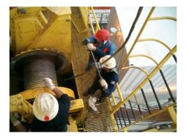
Figure 58 - Secure the rope at the position within the anchor point of the drum
