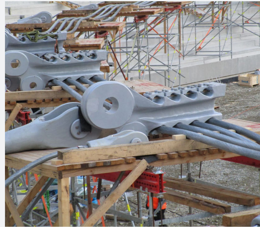
Particular attention is given to ensure all clamp types are designed to an optimum and adequate geometrical shape including rounded edges and with a specific bolt tensioning procedure. NDT tests can be performed on request.
