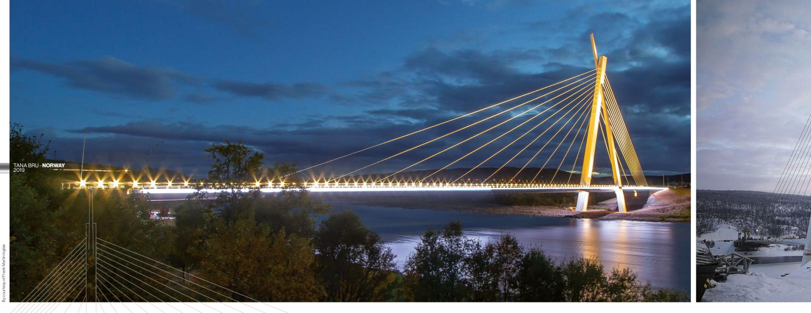
The new cable-stayed Tana Bru Bridge, in Cape North area, is on the main road connecting Norway with Russia. It replaces the old light suspension bridge which was deemed to be structurally deficient and had major weight restrictions in force. The bridge, crossing Tana river, which is famous for quality salmon fishing, has a total length of 260m with main span of 190m.
