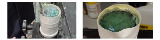
7) The resin must finally cure. A drying time of at least 12 hours is recommended, ideally at an ambient temperature of >15°C. After the resin has dried completely, the protruding rope strands are cut off with a metal saw and the thread of the grouting cone is cleaned of resin residues with sandpaper or a wire brush.
