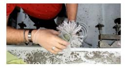
1) The broom base must be moistened with the grouting material step by step until all fibers / twists are soaked.
