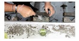
6) The wire bow for working in the resin must have a  $\emptyset \le 3$ mm. Make sure that the fibers are not pushed towards the grouting base.
