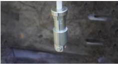
**Unscrew** the grouting cone. The part of the grouting sleeve that is intended for grouting must be free of grease and oil.
